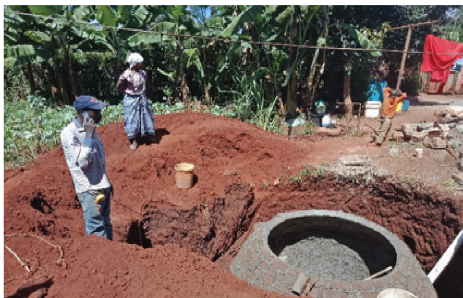
Initial stages of biogas construction in Gatundu North.
